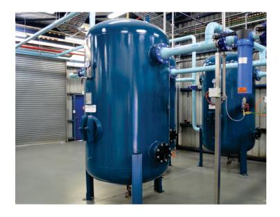
The larger the vessel, the longer the air is allowed to travel through the air receiver and the more condensate that will drop to the bottom to be drained away. Condensate can damage equipment and cause product spoilage.
